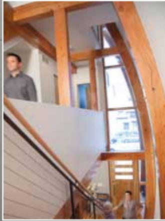
The heavy timber frame used to construct the curved wall adds architectural interest to the home's interior as well.
